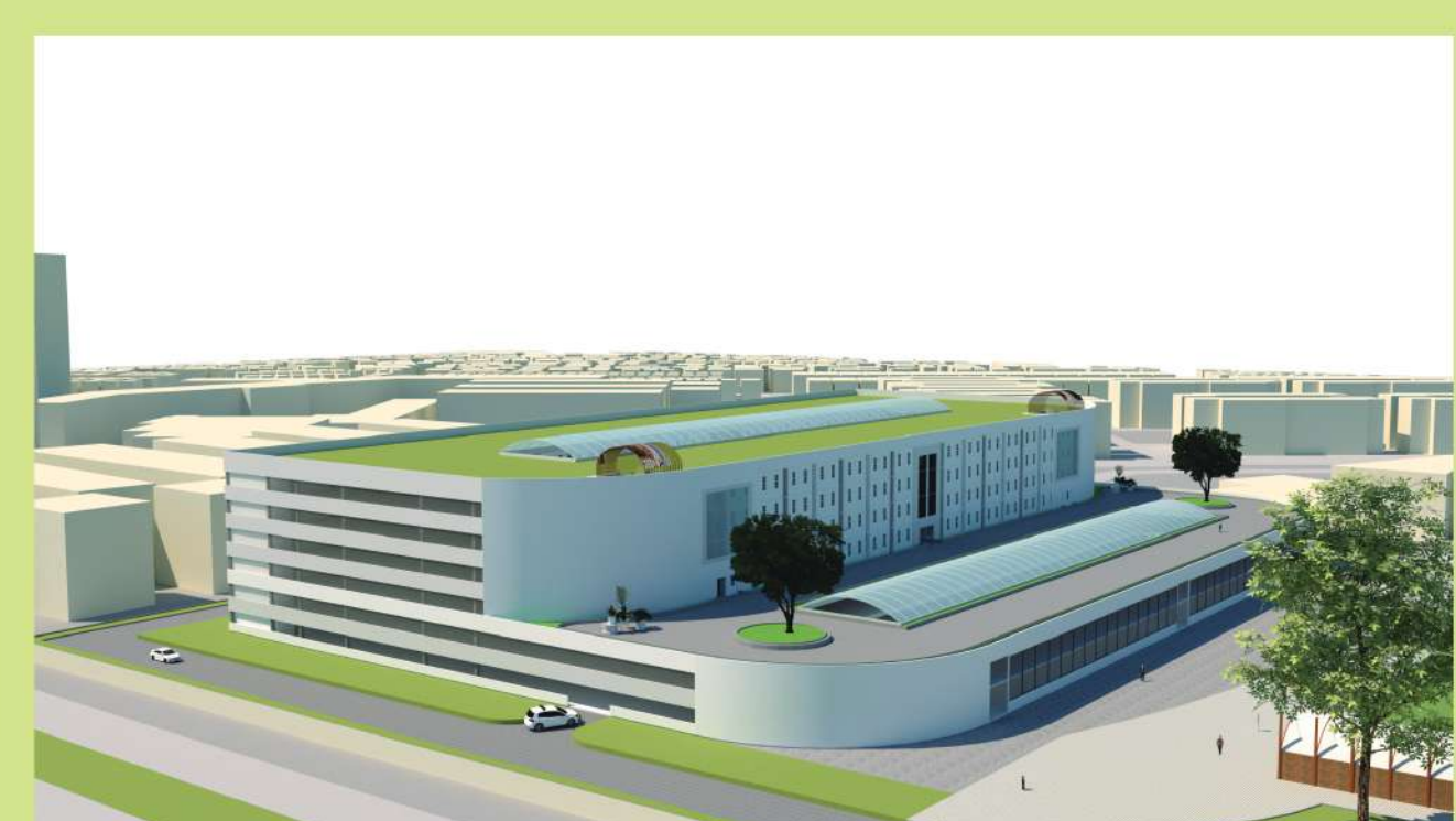
On top of the building is the area for urban farming and the placement of solar panels for energysaving and renewable. The skylight is made of patterned laminated glass so that the light can enter but the heat is blocked
